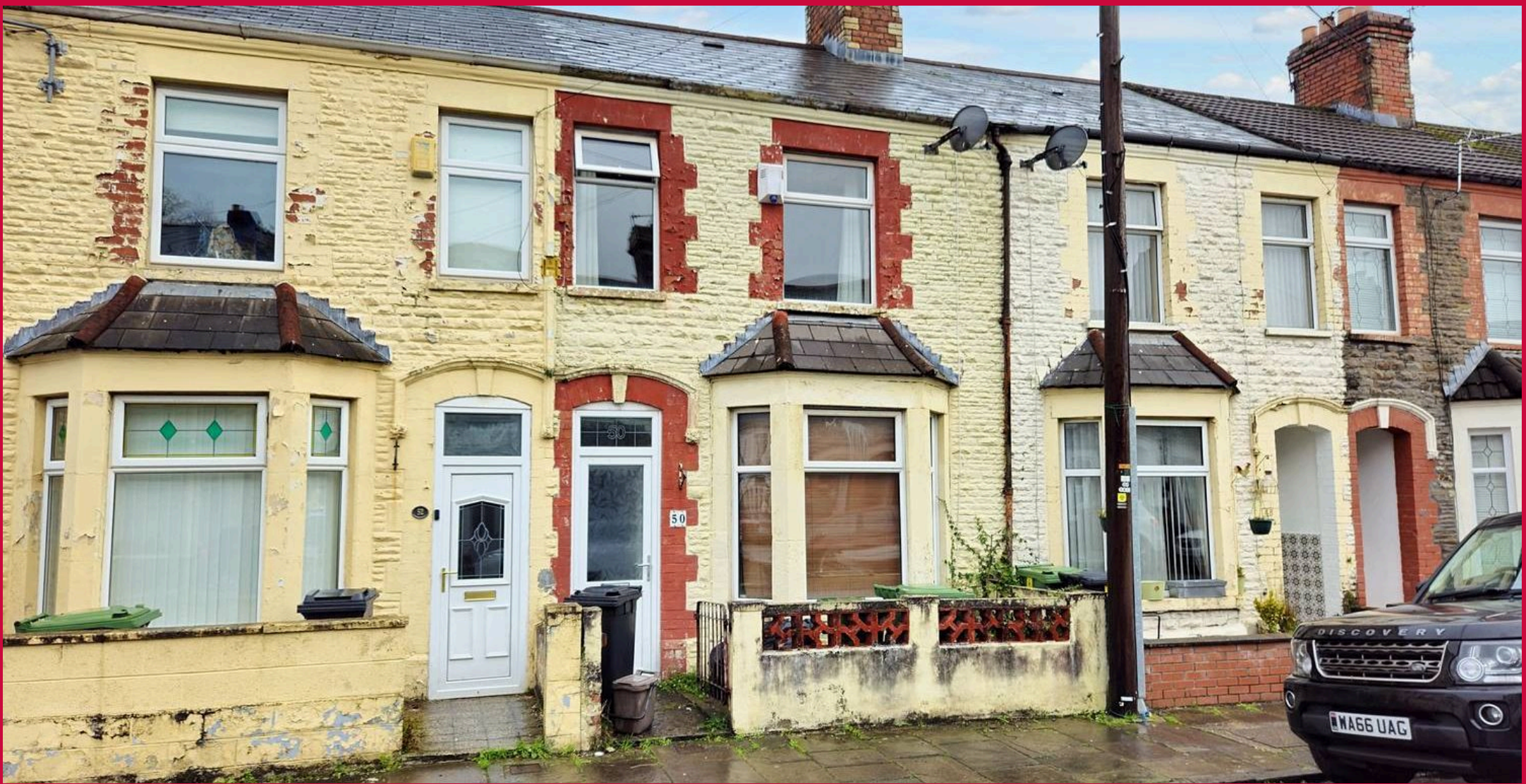
50 Aldsworth Road, Cardiff Cardiff
